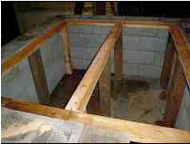
3.1. The form bottom ready for the Hardibacker.
