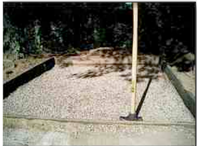
1.2. A gravel or crushed rock bed.
