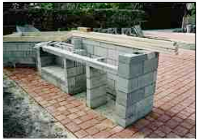
2.6. Stand with cast lintels.
