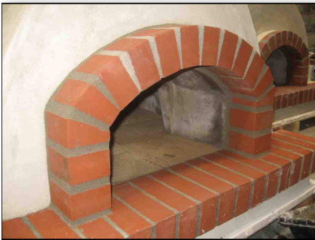
8.1 The Giardino brick arch on a brick oven landing.
