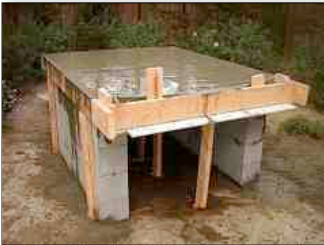
3.6. Structural layer waiting on insulating layer.
