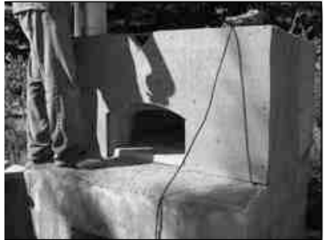
11.4. Attach concrete board.
