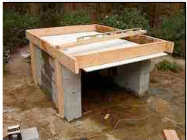
3.3. Hardibacker and form set in place.
