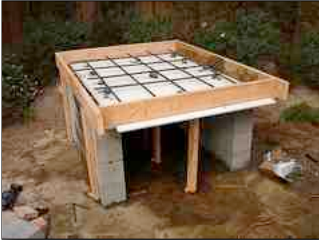
3.4 Rebar set in center of the concrete pad.
