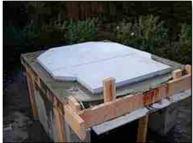
3.7. FB Board set in place.
