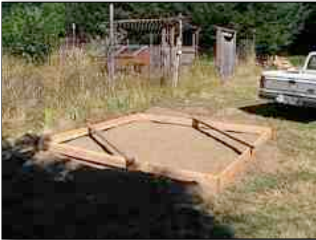
1.7. 2"x4" studs hold the form square and plumb.
