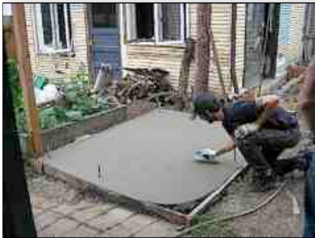
1.4. The finished foundation ready to cure.
