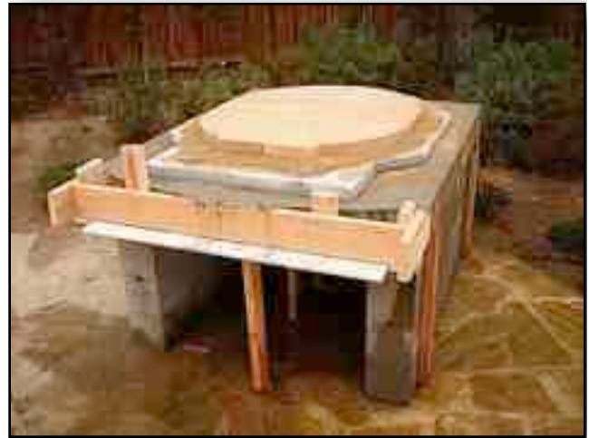
4.2. Set the vent landing level with the cooking floor.
