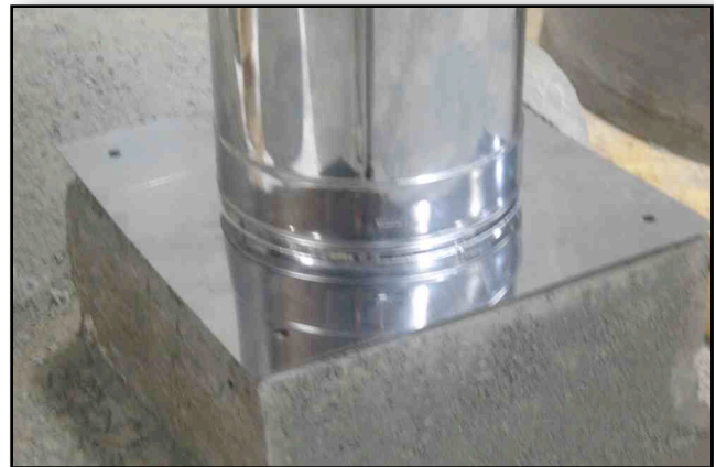
6.3. Attach the anchor plate using concrete screws.
