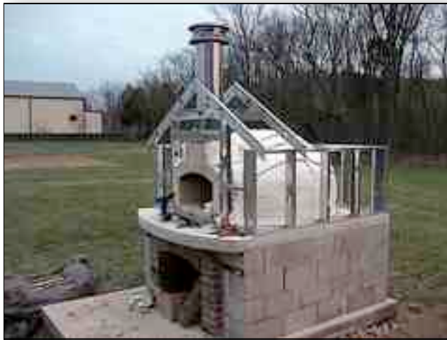
11.3. Metal studs and a gabled roof.
