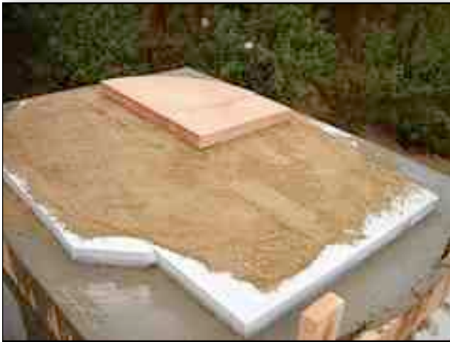
4.1. Set the cooking floor on a thin bed of sand.
