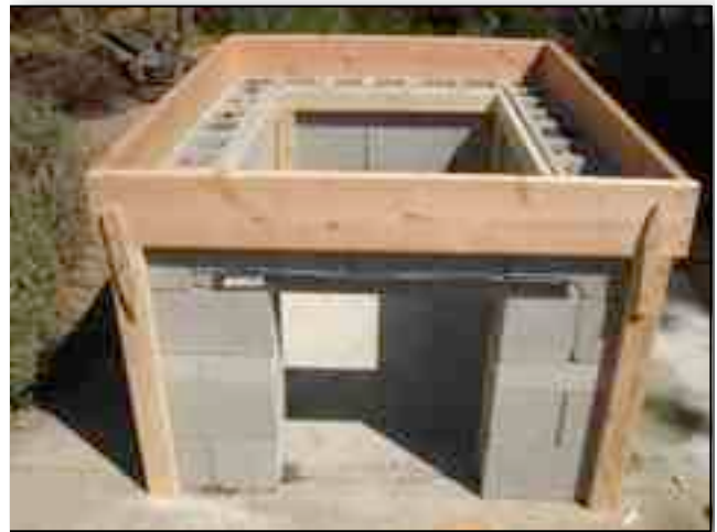
3.2 Form sides held in place with 2"x4" supports.
