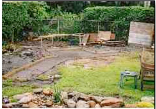
1.5. A complete outdoor kitchen foundation.
