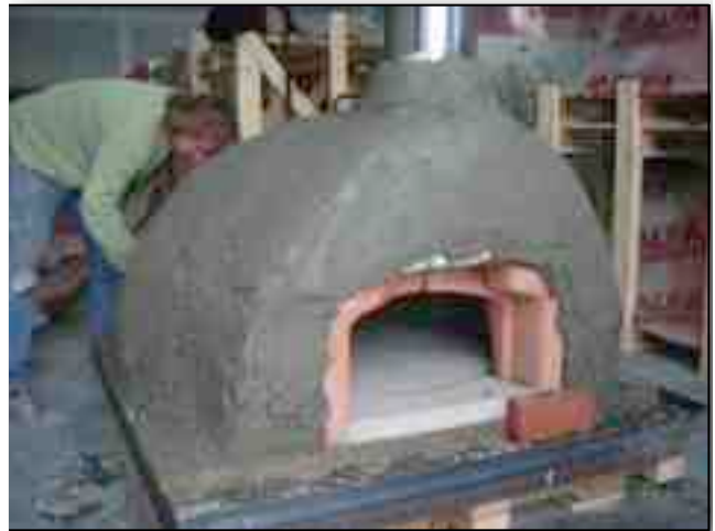
10.3 Rough coat of stucco on wire lathe.
