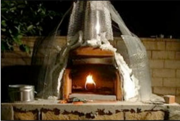
9.3. Rebar and lathe shape the Igloo.
