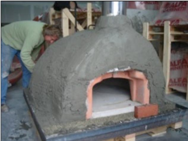
9.4. Rough coat of stucco on wire lathe.
