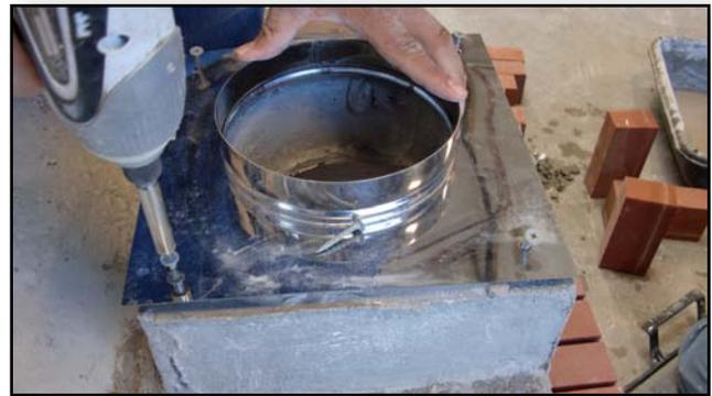
6.5. Screw the anchor plate in place.
