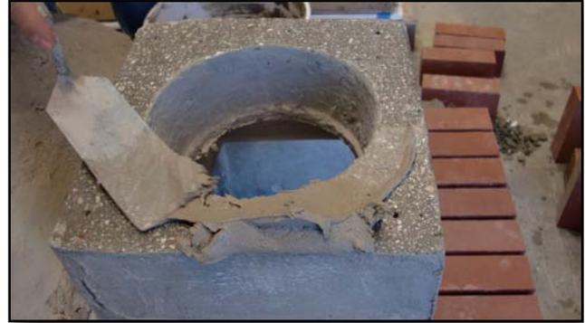
6.4. Apply a bead of refractory mortar.
