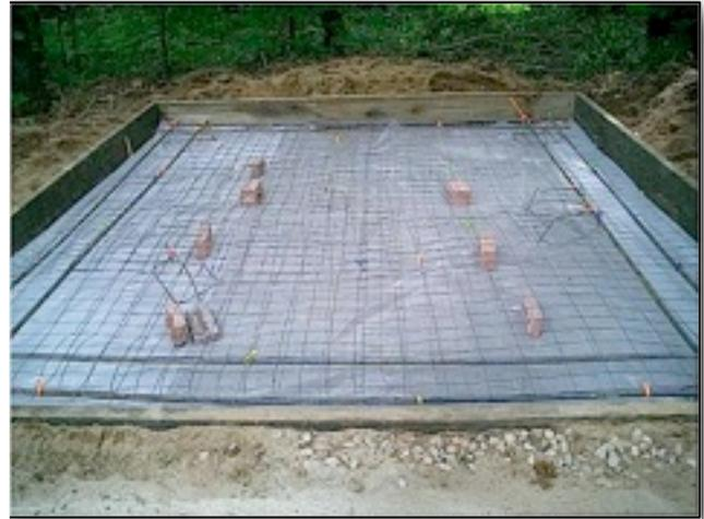
1.1. Framed, lined, with wire mesh and rebar.
